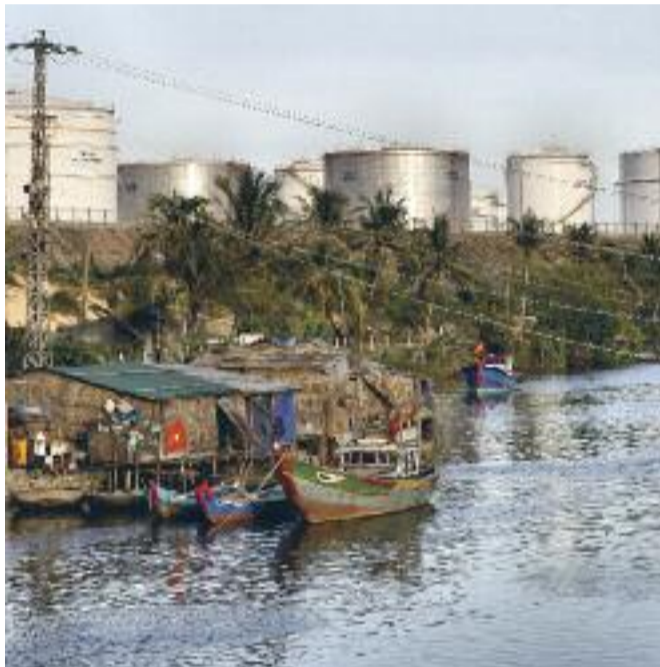
Dung Quat, the first oil refinery in Vietnam, in the Quang Ngai Province. The race to develop energy resources has fuelled growing tensions between Vietnam and China.
