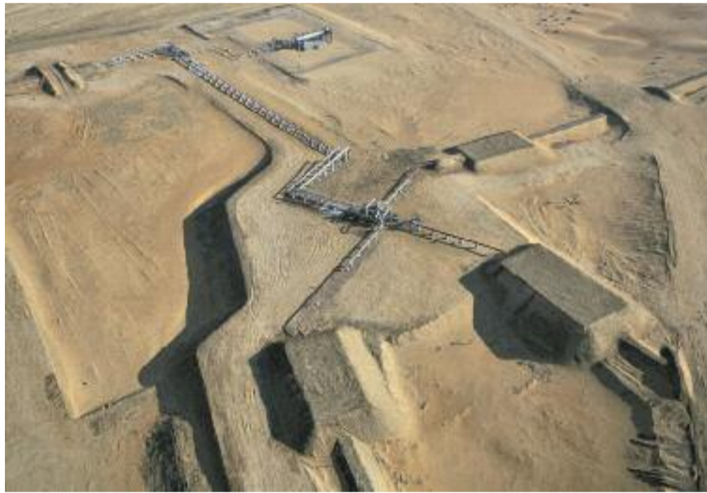
An intersection of the pipelines that lead to the plant for the separation of gas from the oil in the Shaybah field in Saudi Arabia, located in the Rub' Al-Khali desert.
