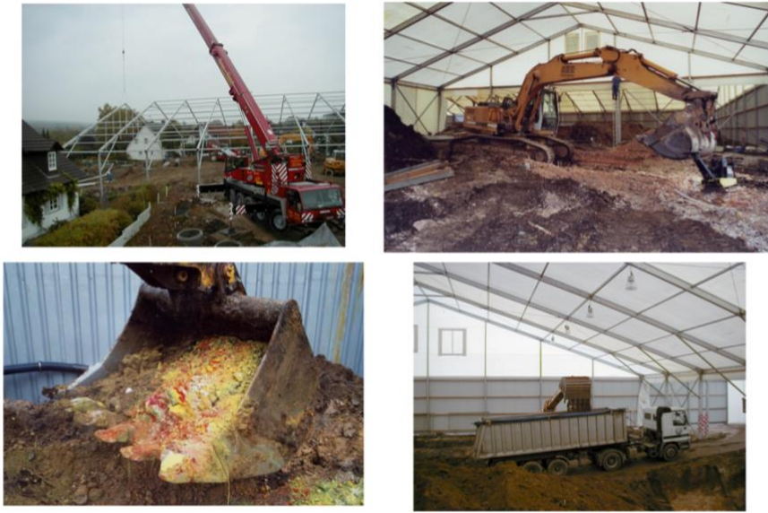
Figure 6-24 Digging & Dumping application case (Source: Professor Petrangeli Papini)
