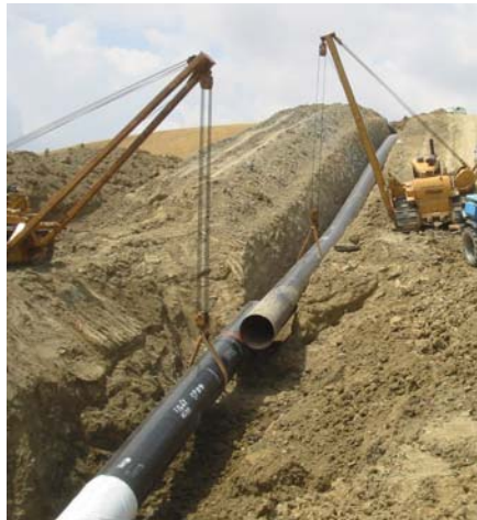
Construction of Enna-Montalbano demonstration tract in Sicily
