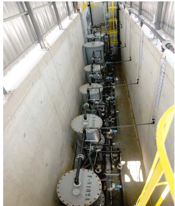
Figure 6: Taranto pilot PRB - the gate containing zeolites and material for As sorption
